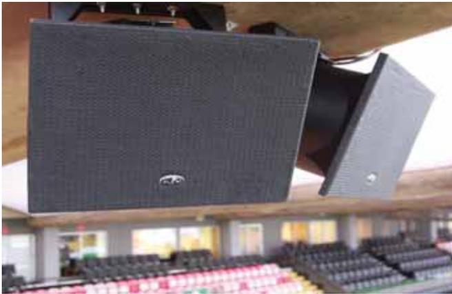
Four D.A.S. BiDriver Plus coaxial horn speakers assist with speech intelligibility
